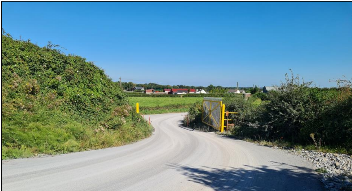
Plate 3-1: View of Access Road and Access Gate
