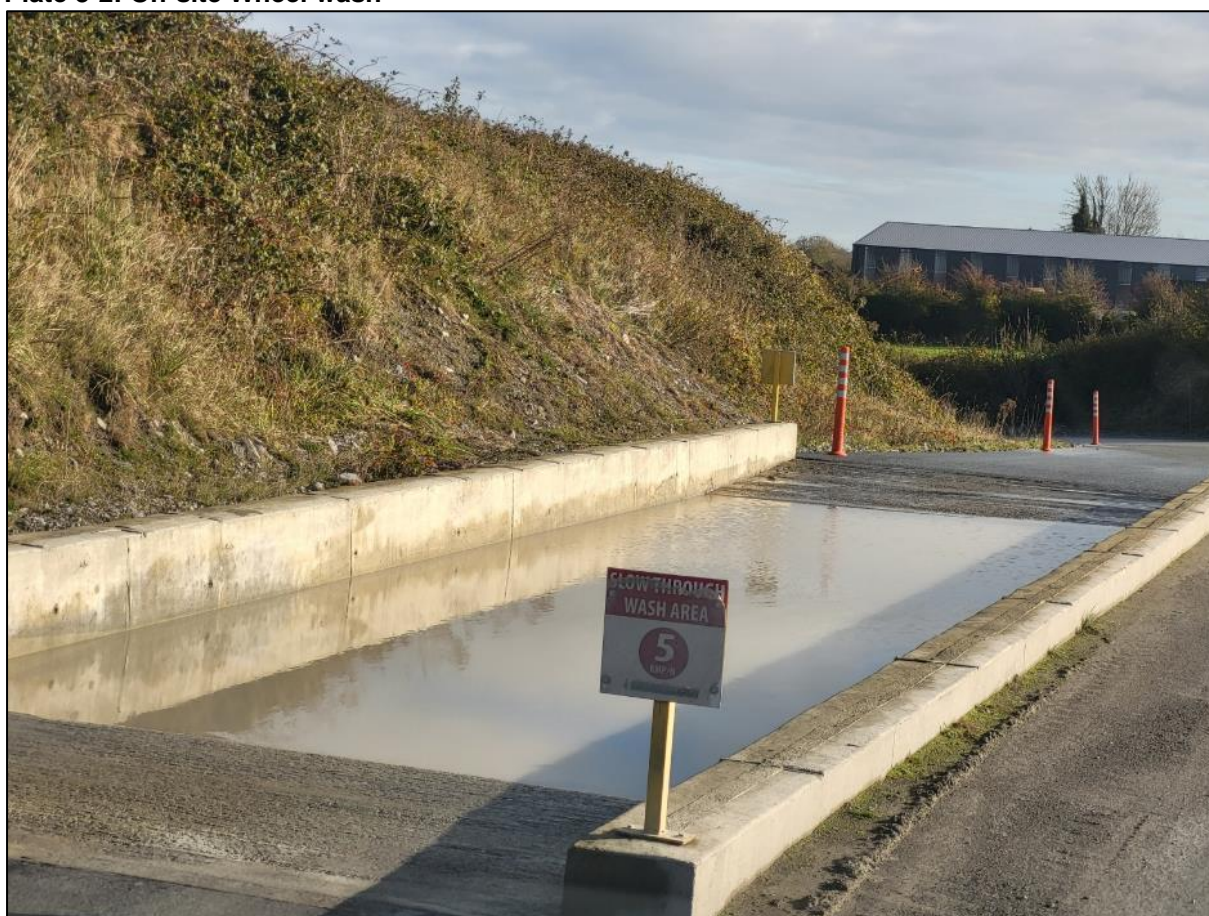
Plate 3-2: On-site Wheel wash
